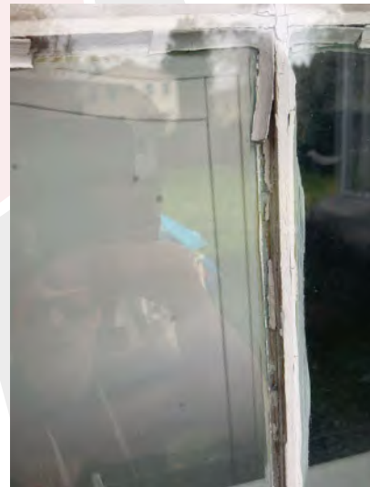
Glazing deteriorated
