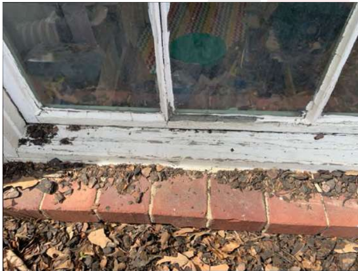
Front left basement window
