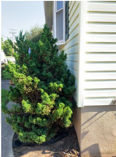
Recommend trimming vegetation away from house
