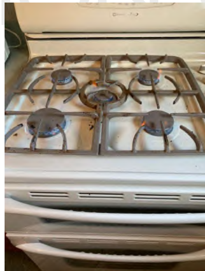
Main floor kitchen stove is missing anti tip bracket
