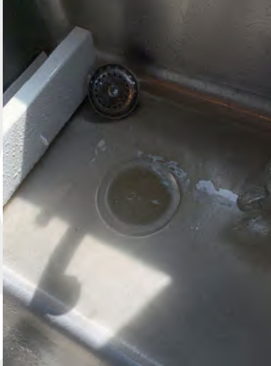
Main floor kitchen sink drains slow
