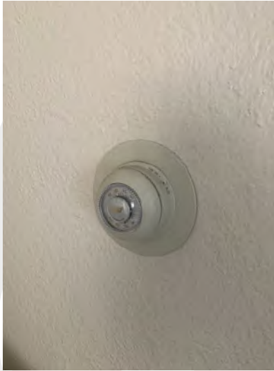
Main floor wall
